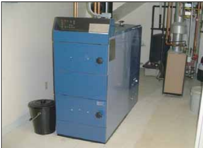
Multi-Heat: Fully automatic stoker boiler with hopper
